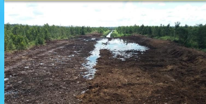
CANAL BACKFILLING TYPE 12 M (LENGTH 250 M)
