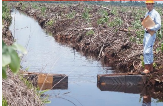
AUTOMATIC WATER LEVEL REGULATOR IN A CONCESSION AREAS (PULP WOOD PLANTATION)
