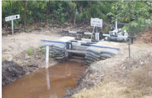
AUTOMATIC WATER LEVEL REGULATOR IN A CONCESSION AREAS (PULP WOOD PLANTATION)
