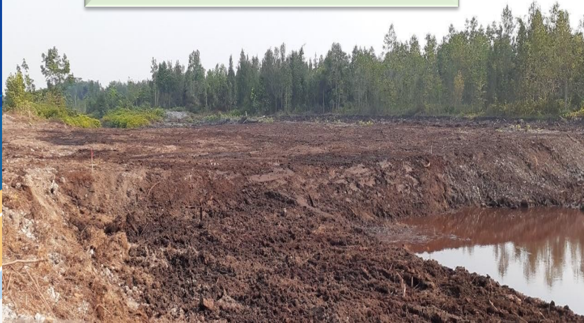
CANAL BACKFILLING TYPE 15 M (LENGTH 250 M)
