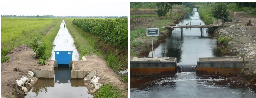
Figure 1. Some models floodgates (flapgate and stoplog / dignity) swamp area in South Sumatera and Central Kalimantan (Doc EdyHarsono and M. Noor)
